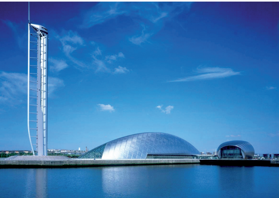
Science Centre Glasgow Foto bdp architects
